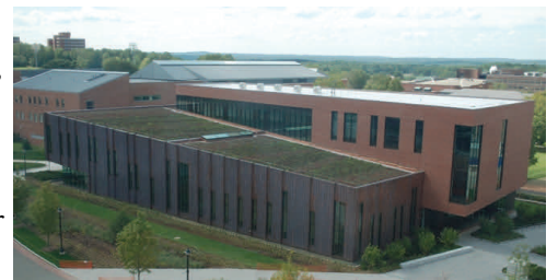
UConn's new Classroom Building on the Storrs campus bodes many environmentally conscious features including a "green roof" and efficient fixtures that reduce water consumption by approximately 48 percent.
